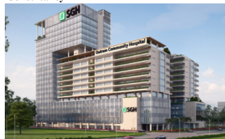
Outram Community Hospital (DBB) (Construction On-Going) Arup: Structure
