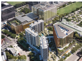
Paya Lebar Quarters (D&B) (Construction On-Going) Arup: Structure + Consultancy
